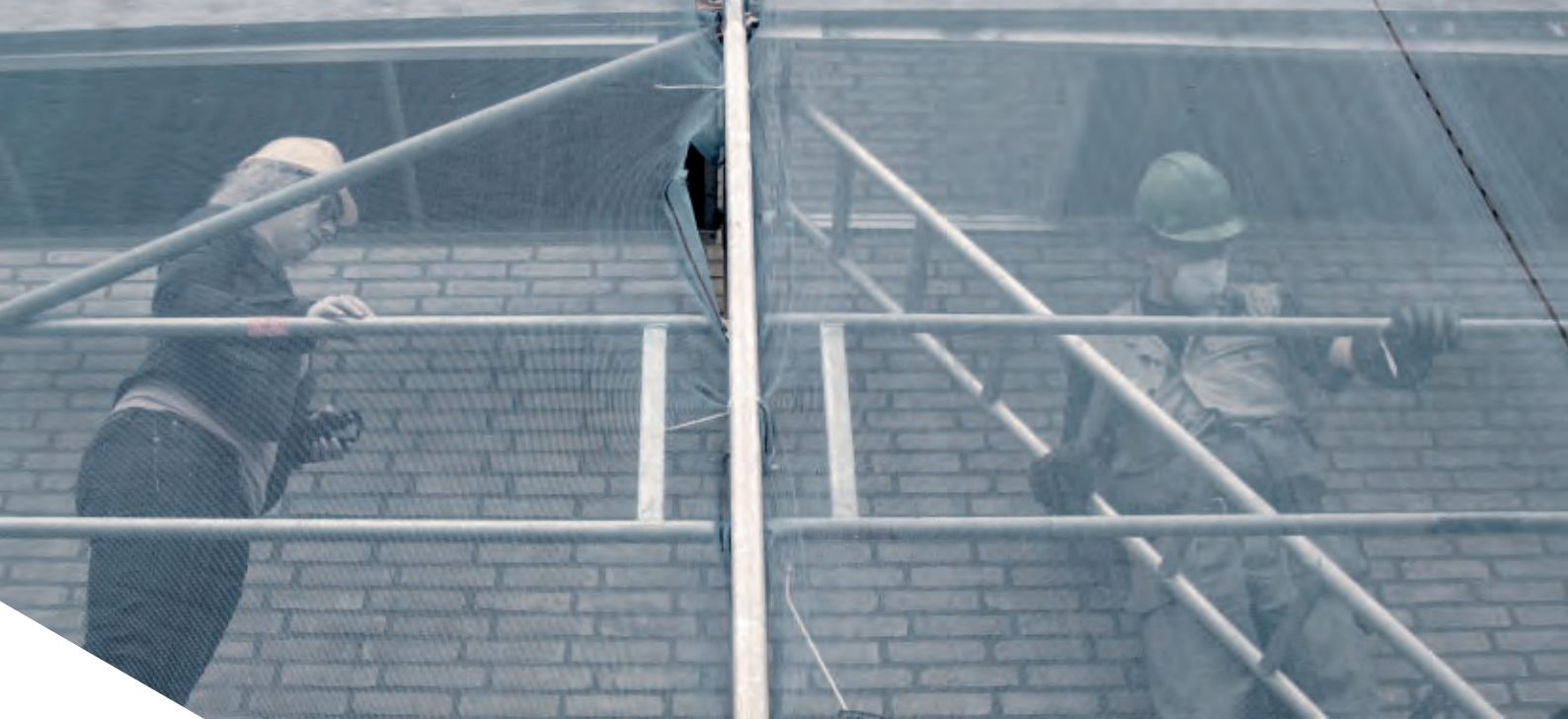
Cindy Bekker (left) is measuring the exposure to nanoparticles during the spray coating of a building facade.
